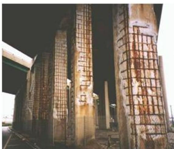
**Figure 1: Bridge Columns Damaged by Corrosion of Reinforcing Steel**
