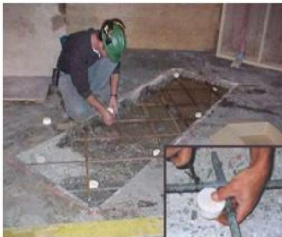
**Figure 2: Alkali-Activated Discrete Galvanic Anode Installed For Localized Protection**
