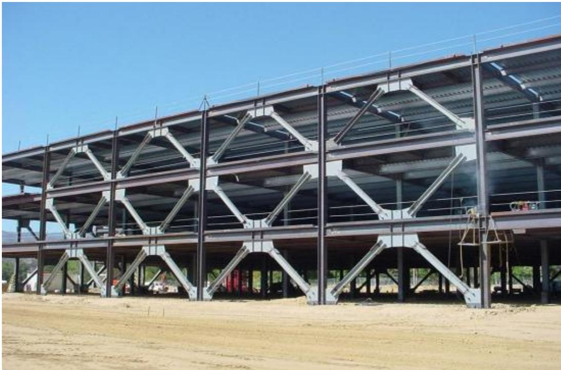
Fig 3: Different concentrically braced frame building Diagonal
